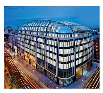
There are several hundred smaller bearings, 110 mm diameter, installed at the first floor level to isolate the exterior triple glazed cladding panels, which are suspended from a steel ring-beam at the level above.
