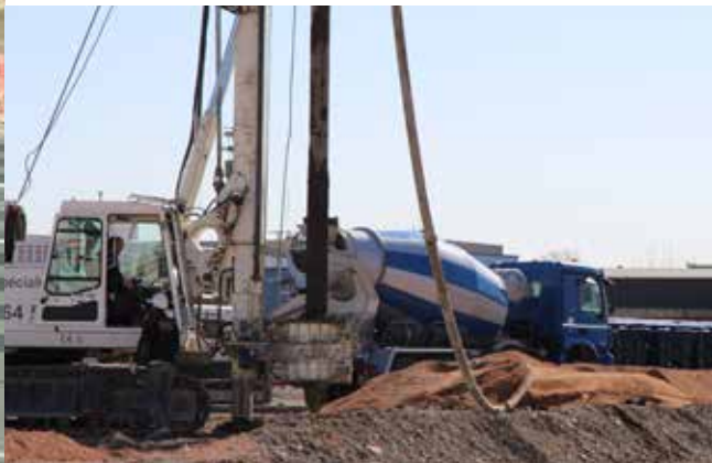
Continuous flight auger piles
